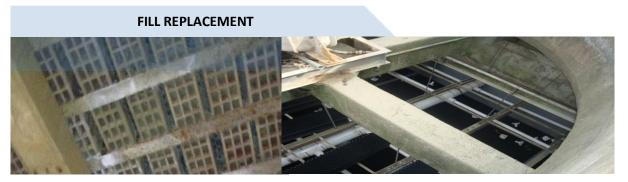
Existing fill was replaced with new PVC fill:15 mil after forming (Brentwood OF21ma-15). Drift eliminators were replaced with PVC Cellular 20 mil. FRP structural shapes were used for fill and drift eliminator support.
