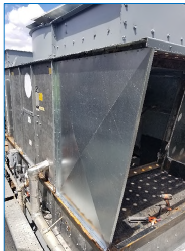
After Sheet Metal Repair
